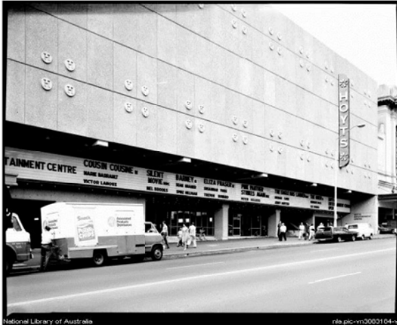
PICTURE 24 – VIEW NORTHWEST ALONG GEORGE STREET TO THE CINEMA
