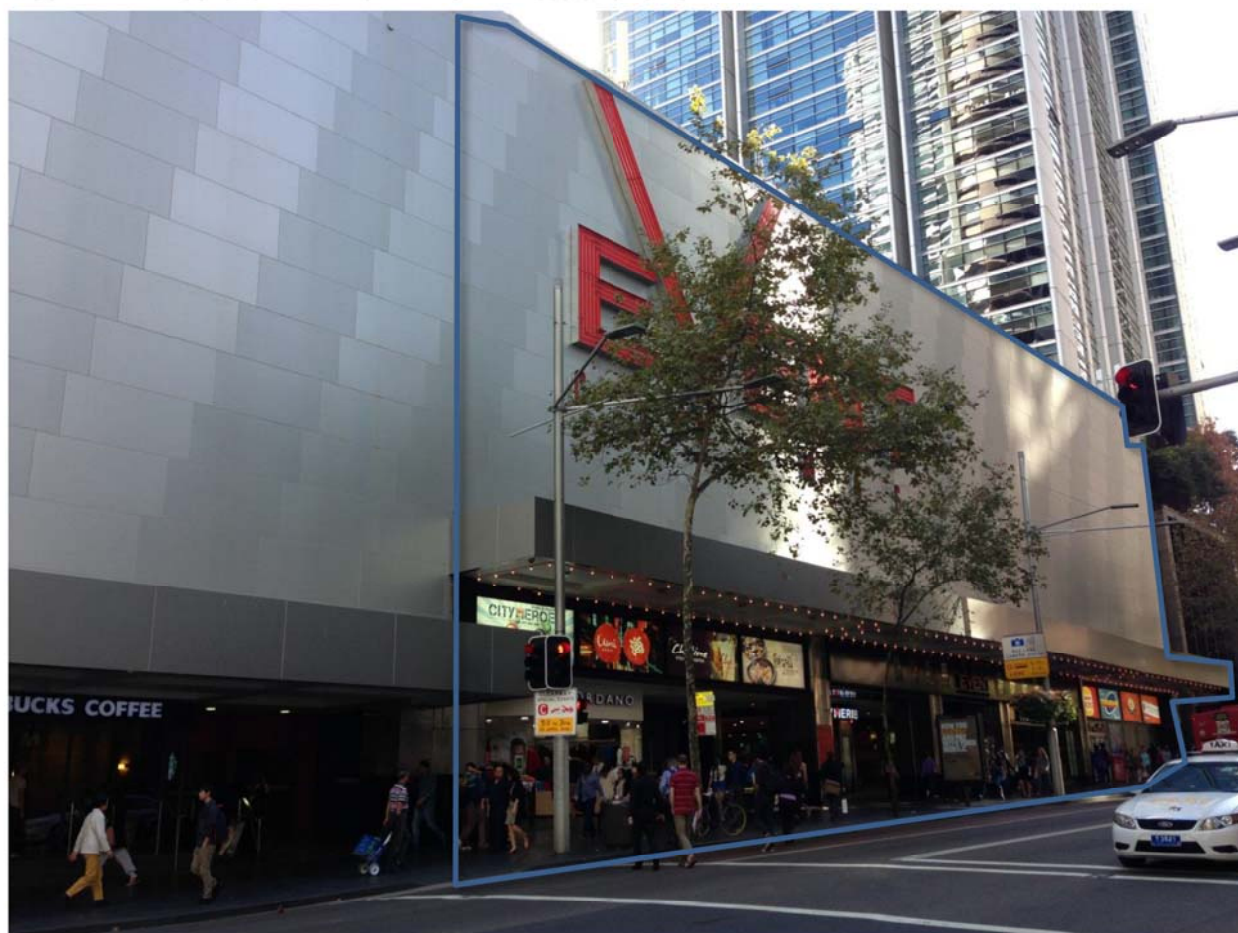
PICTURE 3 – VIEW NORTHWEST TO THE SUBJECT SITE AT 505-523 GEORGE STREET. THE CINEMA TENANCY EXTENDS TO THE NEIGHBOURING PROPERTY AT 525 GEORGE ST, WHICH IS APPROXIMATELY DEMARCATED BY THE LOWER STREET AWNING (APPROXIMATE SITE BOUNDARY INDICATED).
